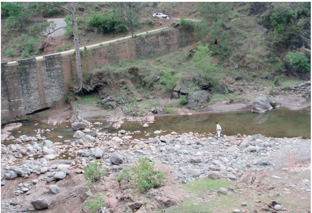
Fig. 14: Angoory bridge spot (East view).
