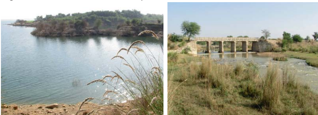
Fig. 73: Right edge of Mangla dam, AJ&K. Fig. 74: Mangla dam out flow stream (Left view).
