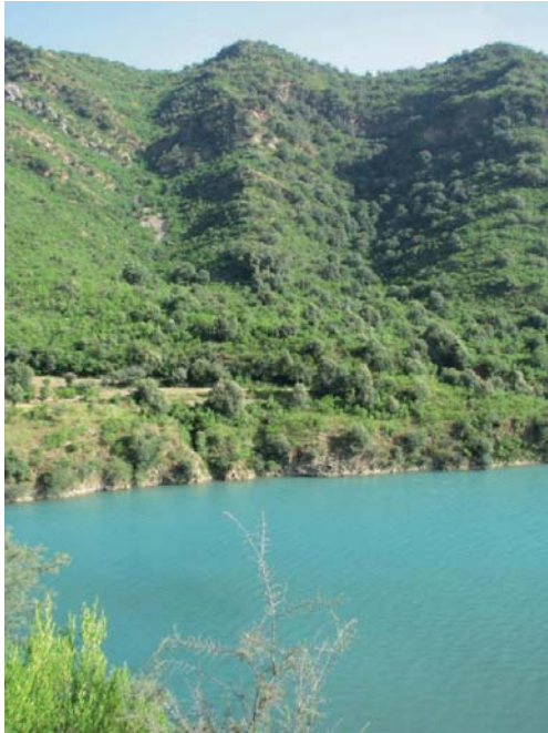
Fig. 68: Rear side view of Khanpur dam at Bhamala.
