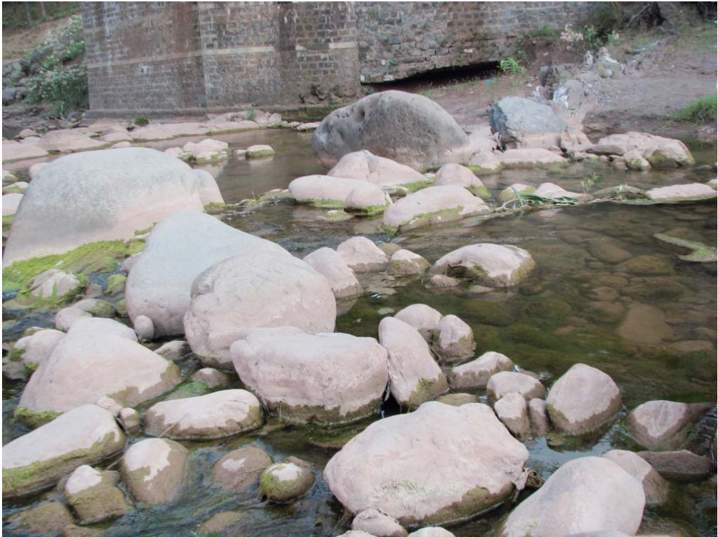
Fig. 13: Angoory bridge spot close up view (East).
