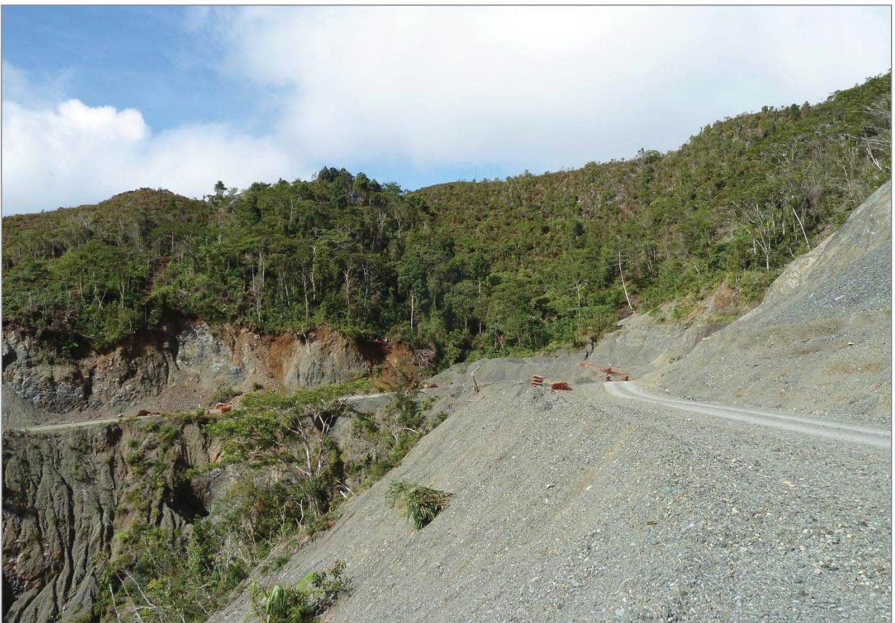
Figure 4c, d. Newly cemented road, cutting the mountain.
