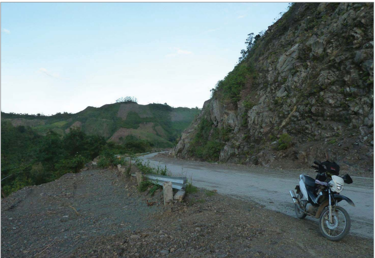
Figure 3a, b. New road connecting Davao del Norte province to Bukidnon province.
