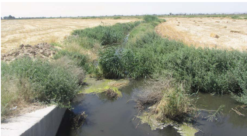
Fig. 11. A concrete canal 3 km south west of Qomroud city, Qom province (Loc. 11).
