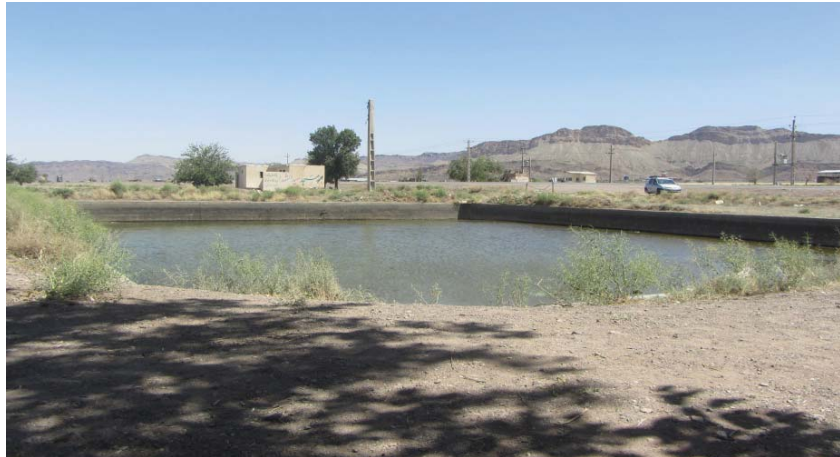
Fig. 8 a. A reservoir at Zanburak village, Qom province (Loc. 7). b. Concrete channels that connect the reservoir of picture (a) to another one.
