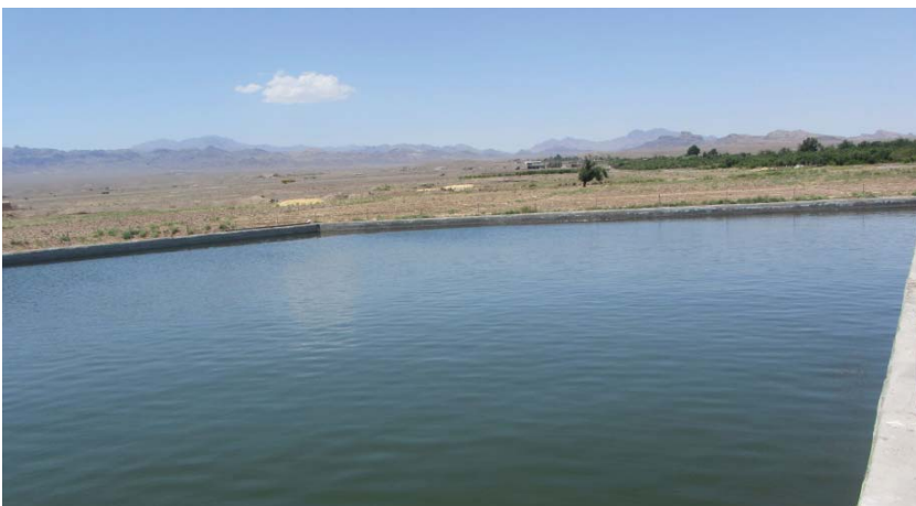
Fig. 5. A reservoir at San San village, Esfahan province (Loc. 4).
